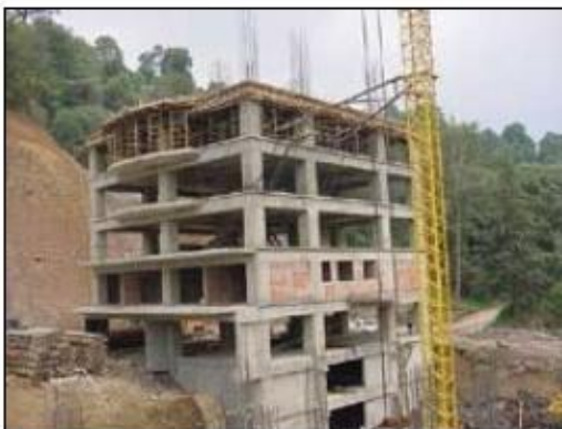
Figure 1. RCC Frame Structures
