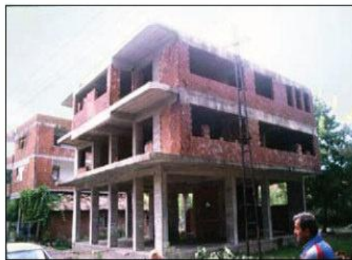
Figure 2. Infill Frame Structure
